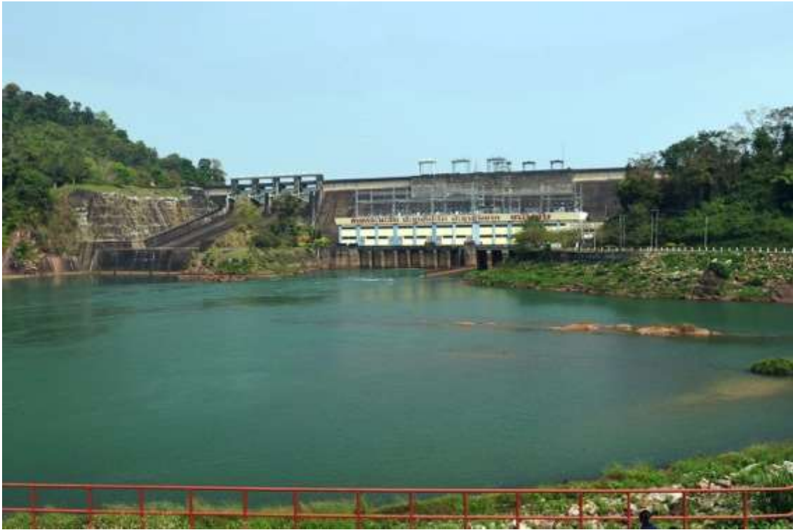
Figure 1 – Downstream of Nam Ngum dam and hydroelectric plant in Lao PDR
