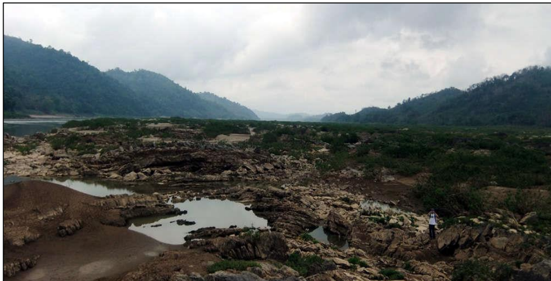
Panoramic View at Upper Dam Site (Look to D/S)
