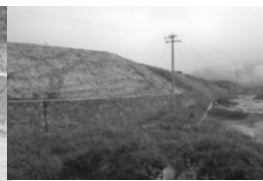
砌石挡墙护 Stone retaining wall at gravel yard
