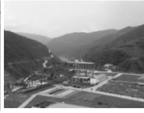
⑥ Construction Site View
