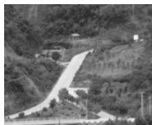
渣场绿化措施 坡 Spoil yard landscaping measures
