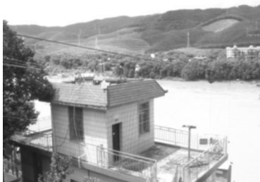
Yunjinghong Hydrological Station
