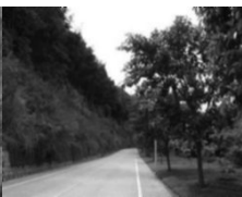
进场公路绿化措施 Accessing road landscaping measures
