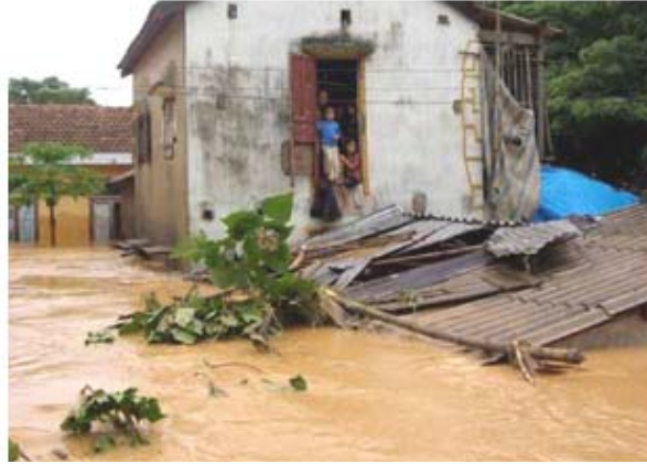
Figure 7.3: Ketsana. Property damage Quang Ngai Province.
